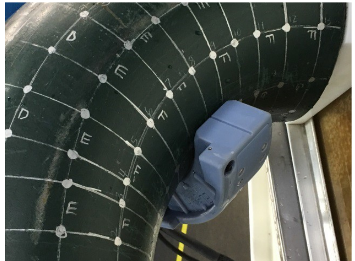
Scanner on elbow intrados
